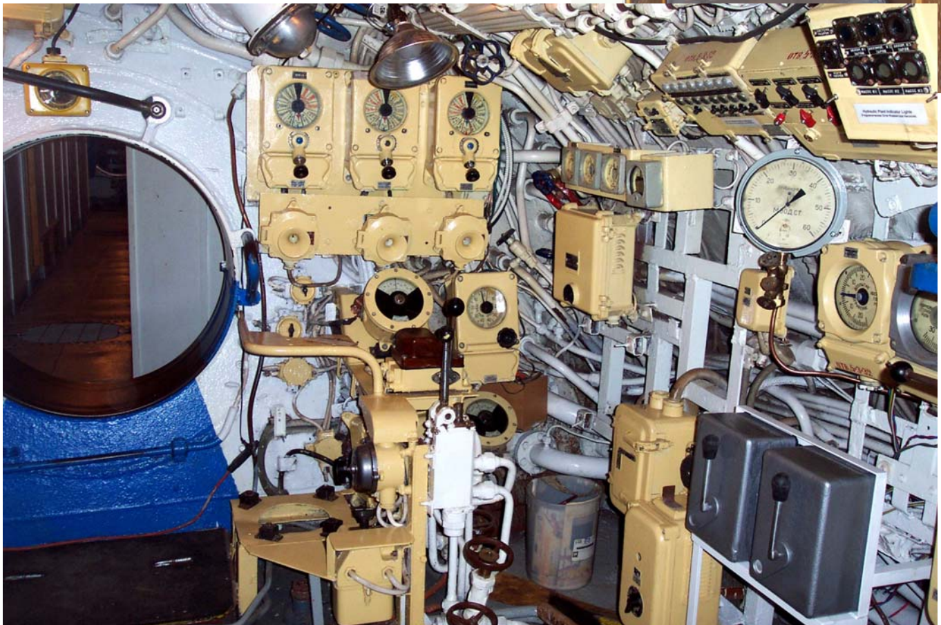
The Control Room with the new bow and stern plane controls and depth gauges (shown on the right side of the photo)
